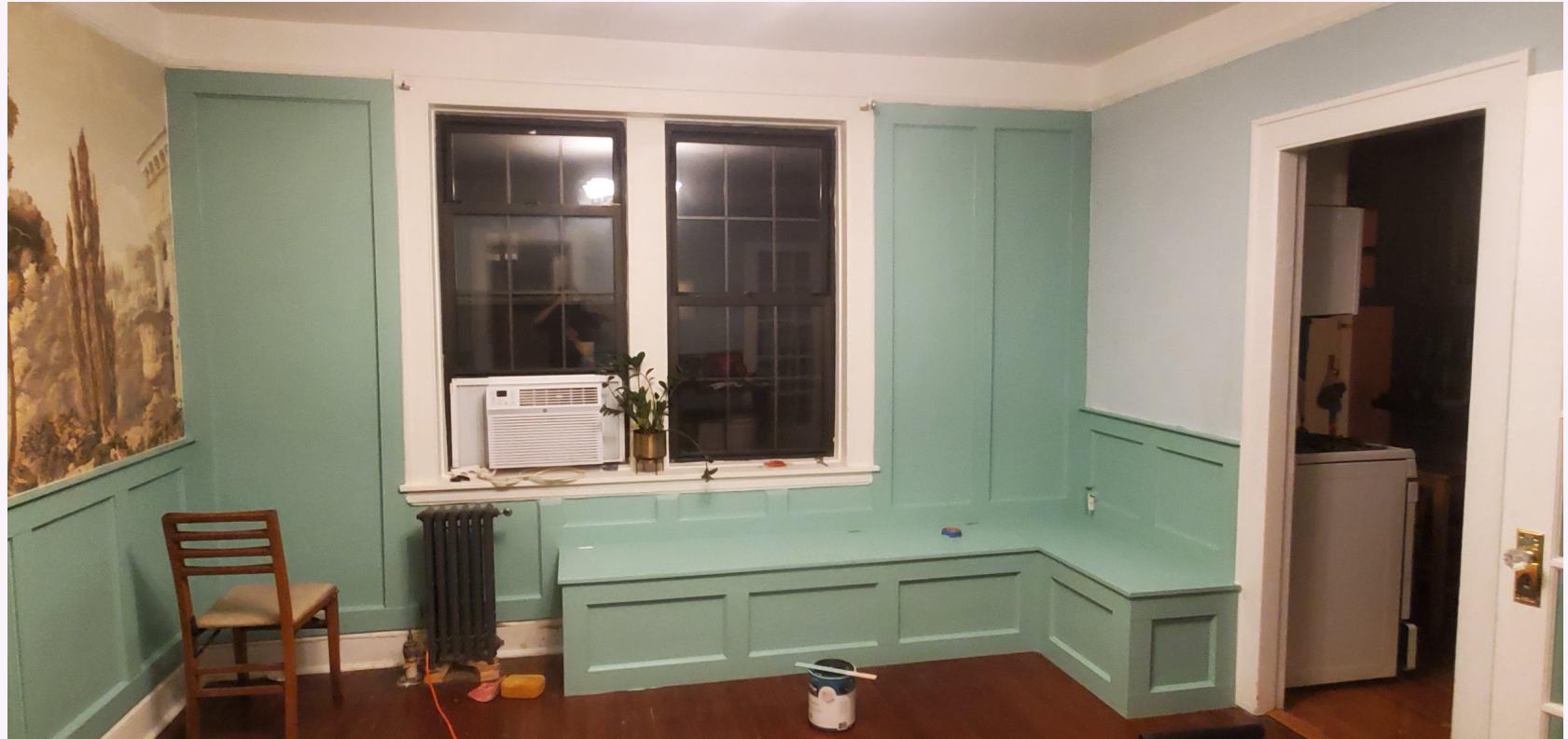
interior: custom millwork, wallpaper, custom upholstery, electrical wiring
